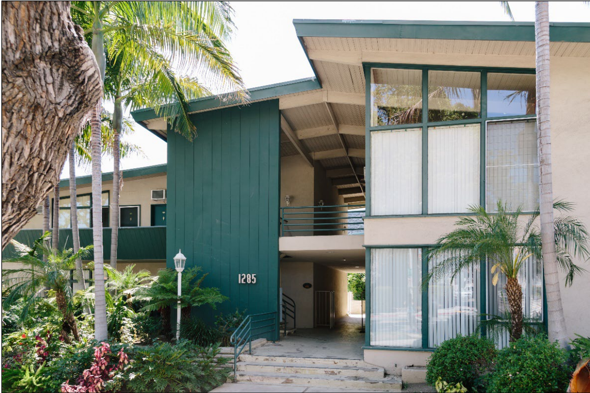
Figure 24: The Fountain Lanai (1285 Sweetzer Avenue), 2015. This building is a designated example of the Mid-Century Modern style that is individually listed as a West Hollywood Cultural Resource (Tony Coelho, City of West Hollywood).
