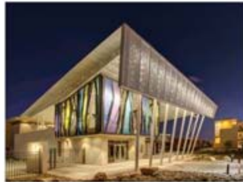
Figure 4-7. A long-term care facility in an LZ-3 area: well-shielded lighting—no direct uplight. (Image courtesy of David Roederer)
